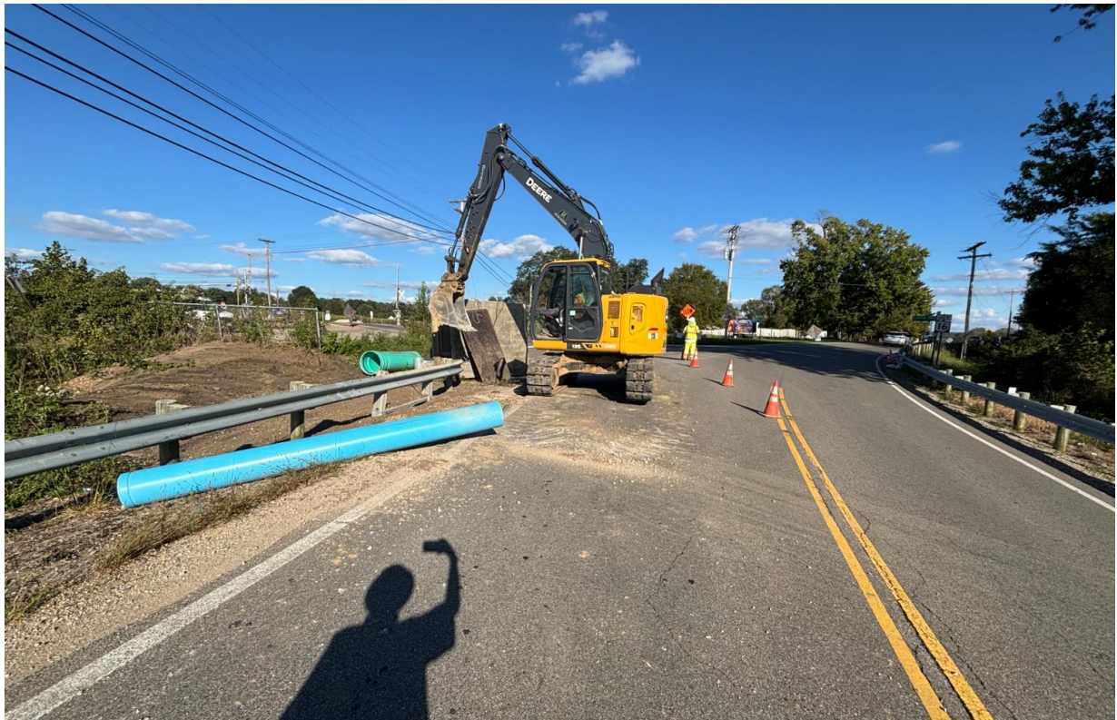
MARNE Rd. repair to large unknown clay storm pipe near Licking Valley Rd intersection
