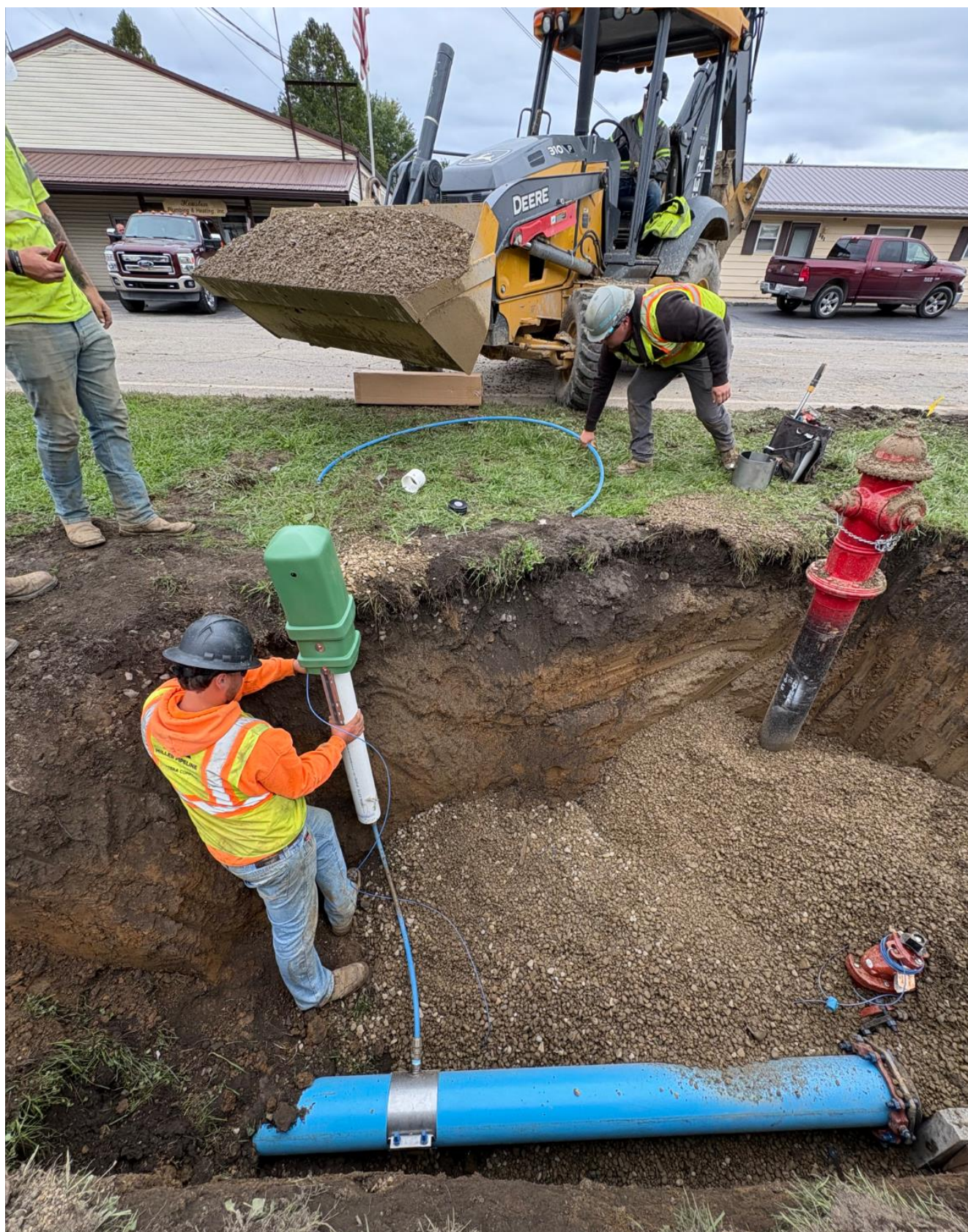
Water testing box install on MONTGOMERY Rd. 1 of 4 Phase I install locations.
