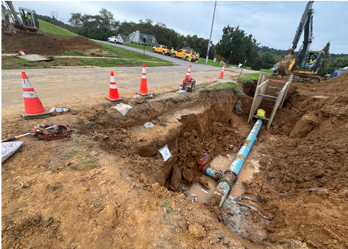
MARNE Rd. repair to large unknown clay storm pipe near Licking Valley Rd intersection
