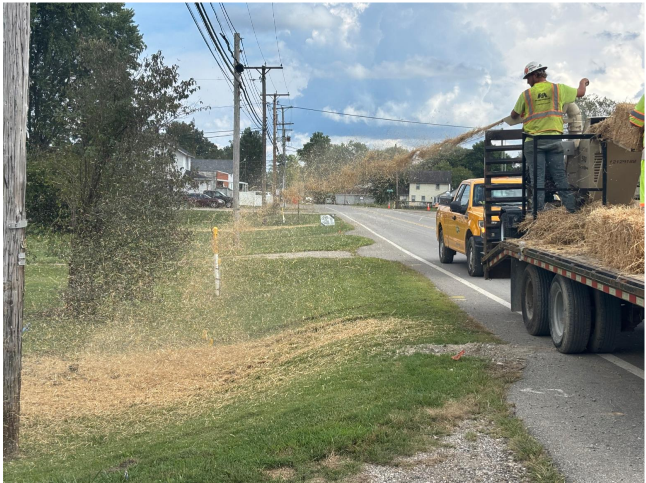
Placing seed and straw to stabilize daily water service box install areas on MARNE Rd.
