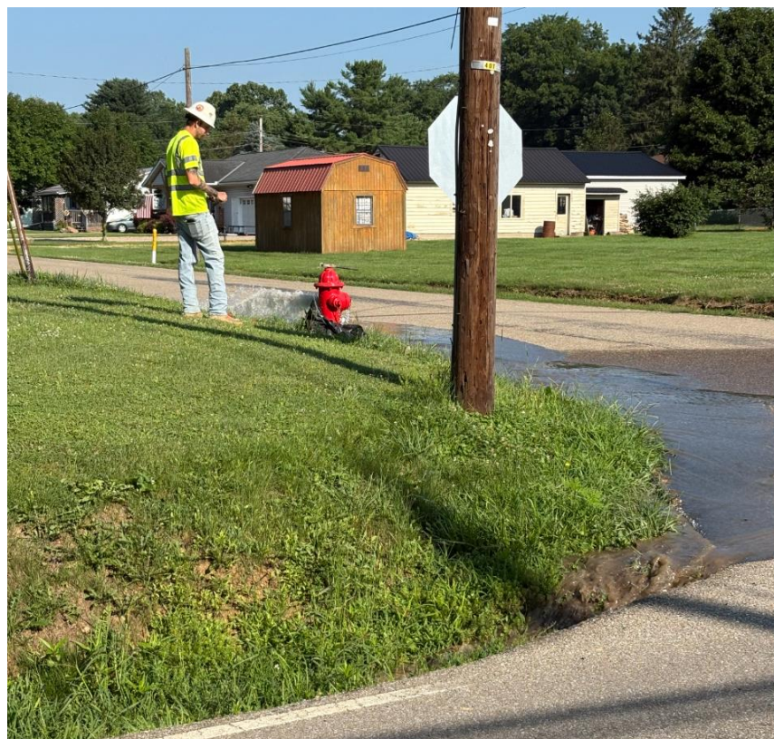
MONTGOMERY Road flush and pressure testing N side of railroad
