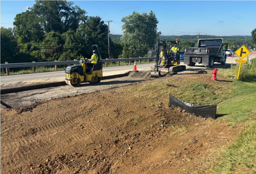
Pavement repairs on Licking Valley Rd. last full week of June. Rough grading along school frontage complete and erosion controls in place ready for seed and straw stabilization
