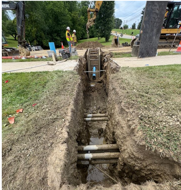
Looking West at 12" watermain that will go under located electric and communication conduits to Primary School
