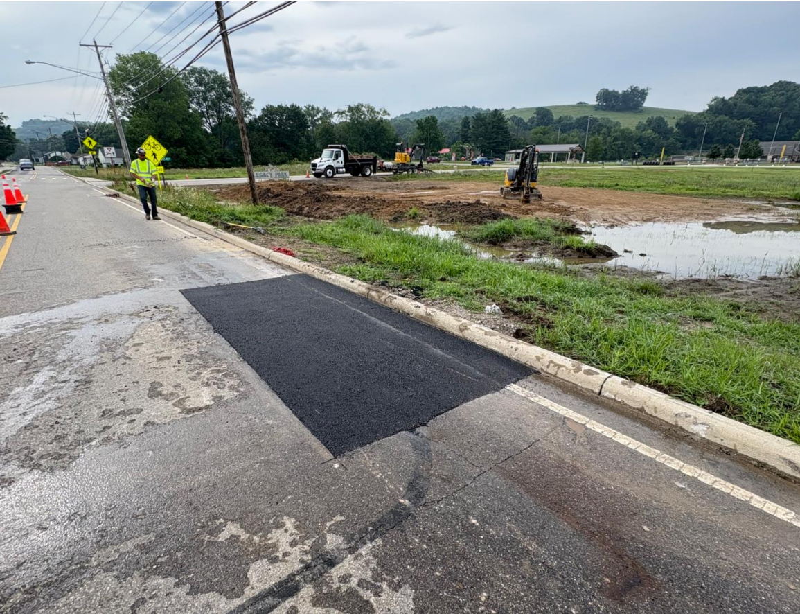
Pavement repairs on Licking Valley Rd. last full week of June. Rough grading along school frontage complete and erosion controls in place ready for seed and straw stabilization
