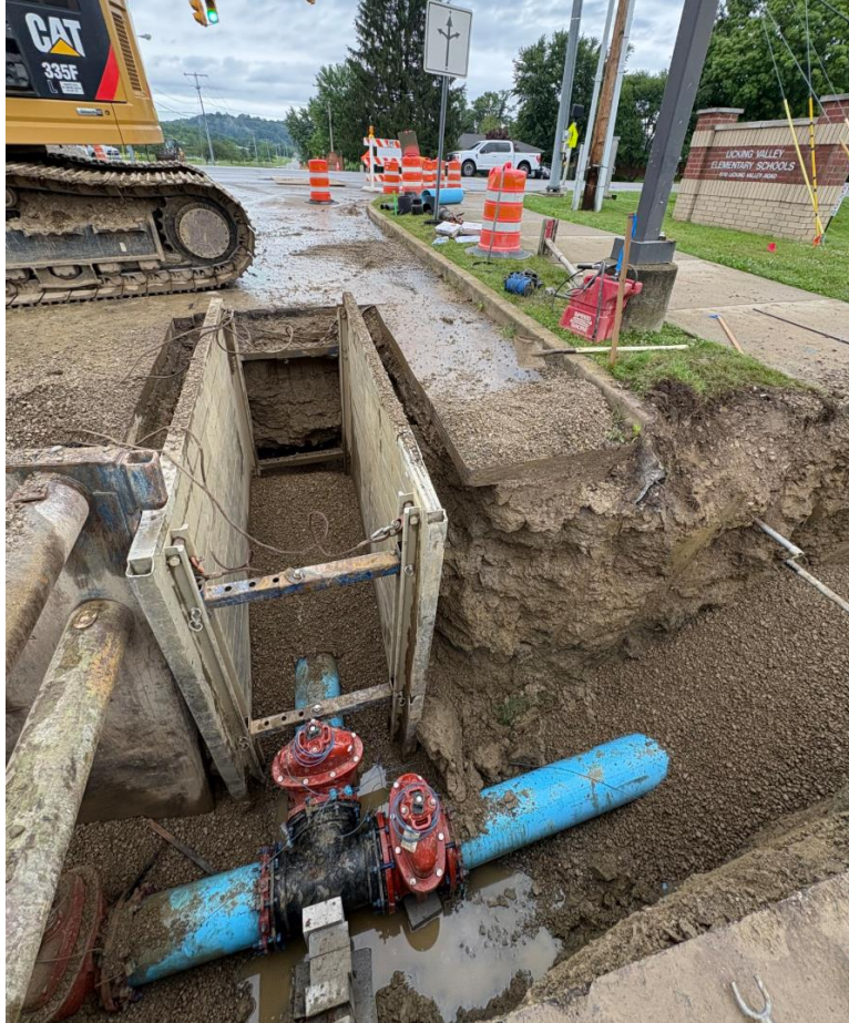
Looking West at 12" watermain that will go under located electric and communication conduits to Primary School
