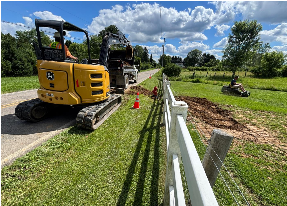
Restoration, grading and topsoil follow up on SWANS Rd.
