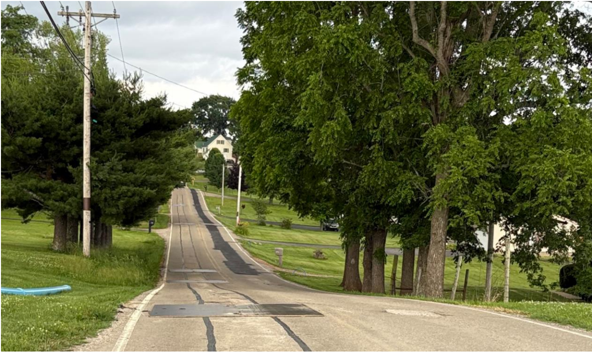
Preparing DARLA for full-depth pavement replacement
