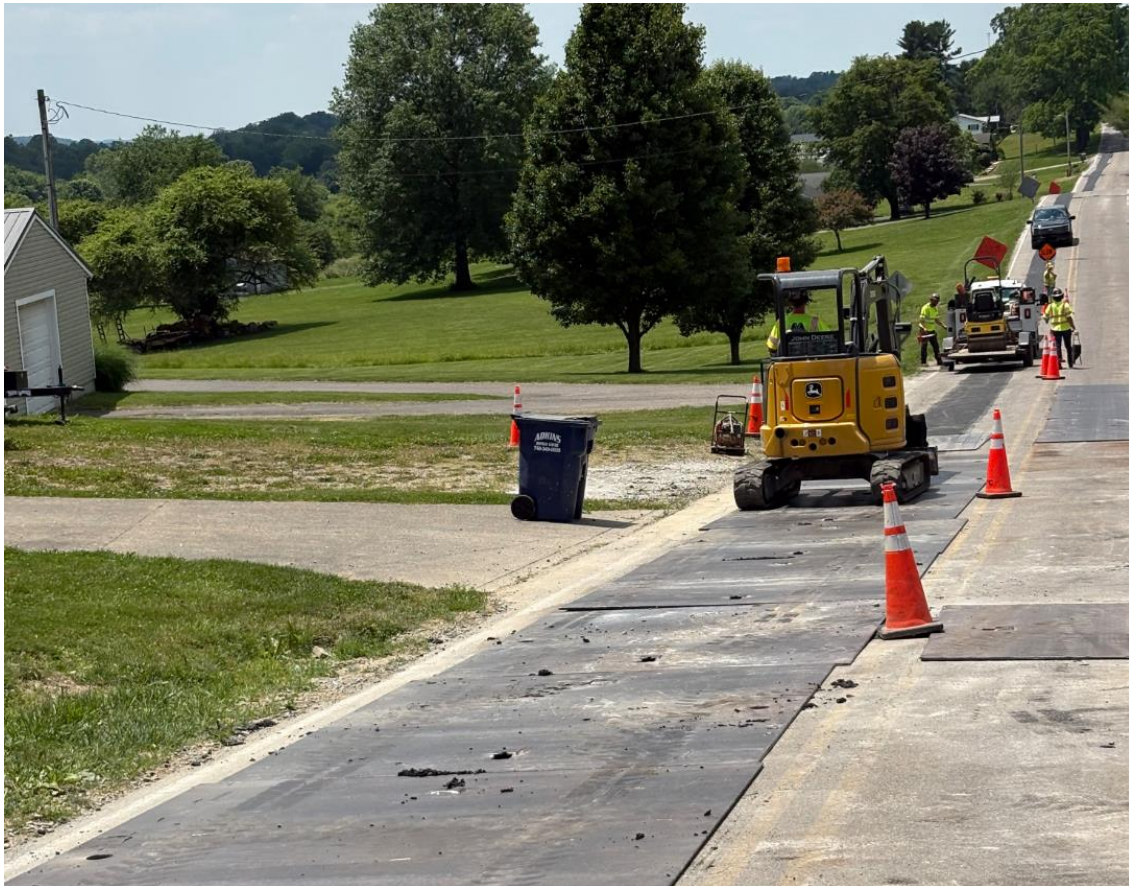
Bolen Rd. pavement replacement crew
