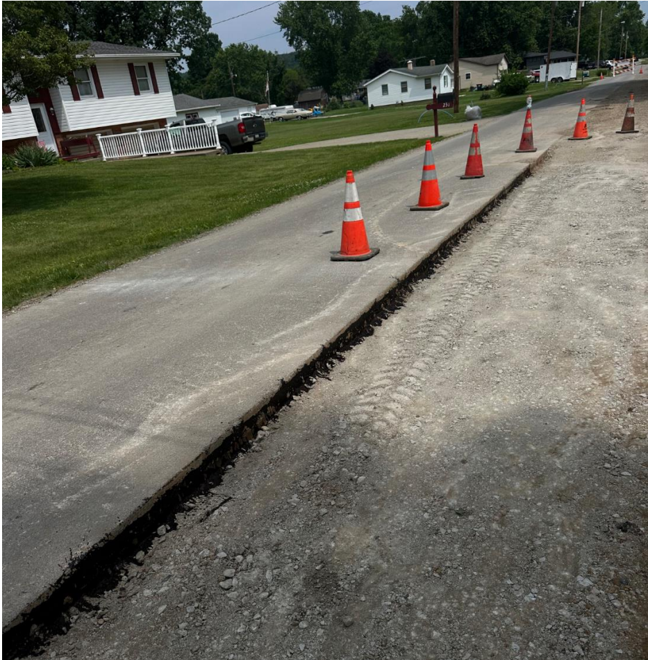
Preparing DARLA for full-depth pavement replacement
