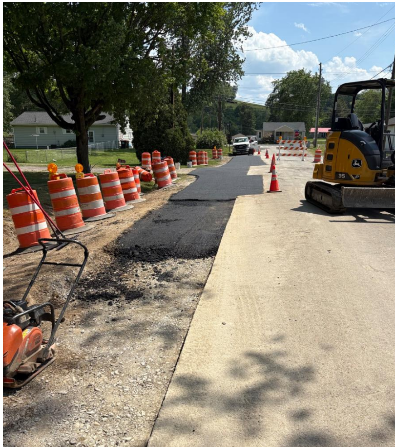
Process of pavement repairs on DARLA
