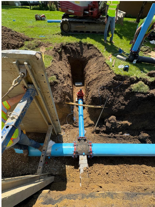
Typical hydrant install on 12" Watermain with a 12"x6" tee. Tee, valve, hydrant block support to native soils.
