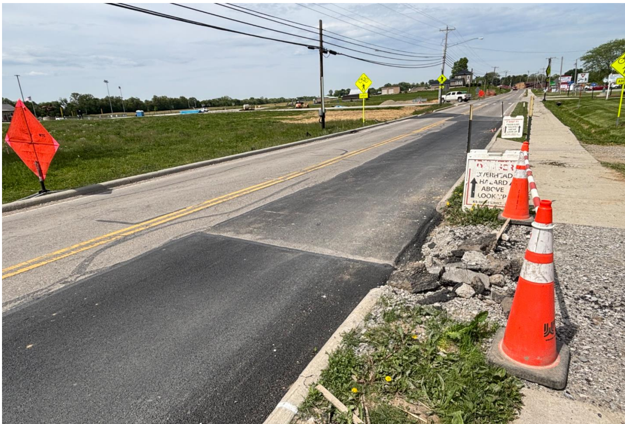
Asphalt Pavement Repairs over 12" Mainline on W HIGH are caught up, maintenance of traffic warning devices in place, sidewalk backfilled level to maintain pedestrian access
